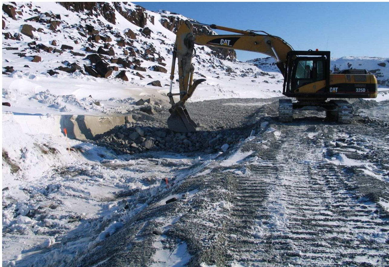
Photo 3: Placing second lift of ROQ ~ Sta 5+30.325 excavator was down for much of the day.
