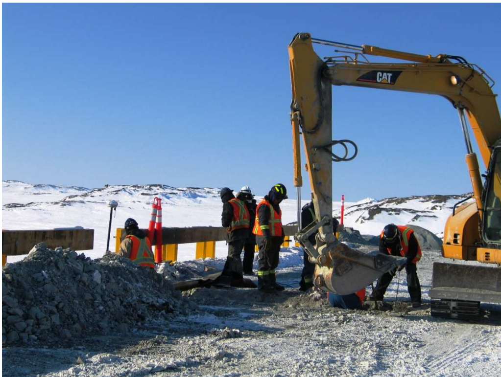
Photo 5: Installing thermister SRK-DWB2. Excavator is filling hole. Surveyor is surveying bedding layer.
