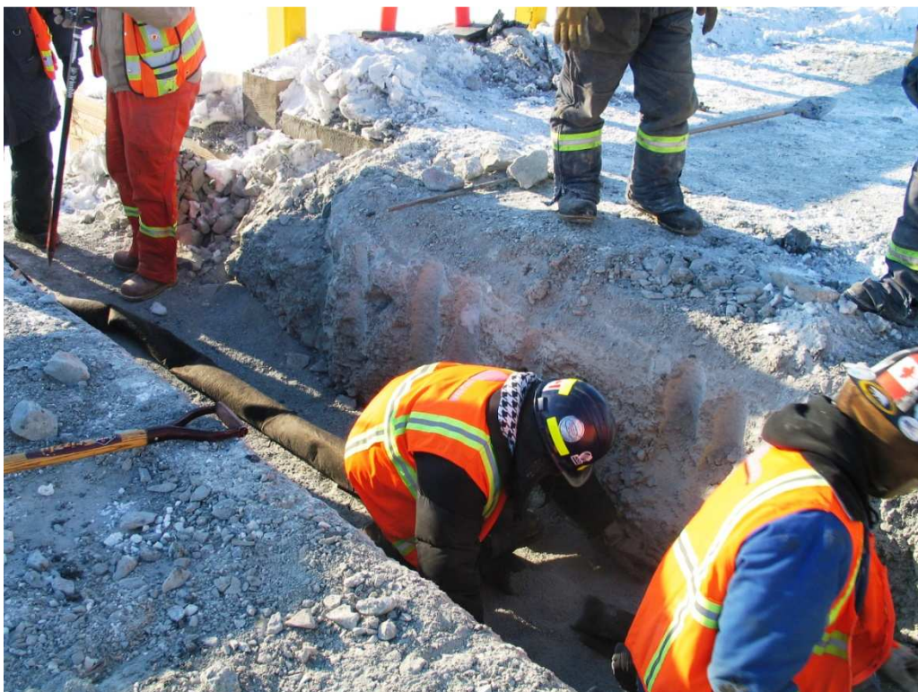
Photo 6: Cable wrapped with geotextile.
